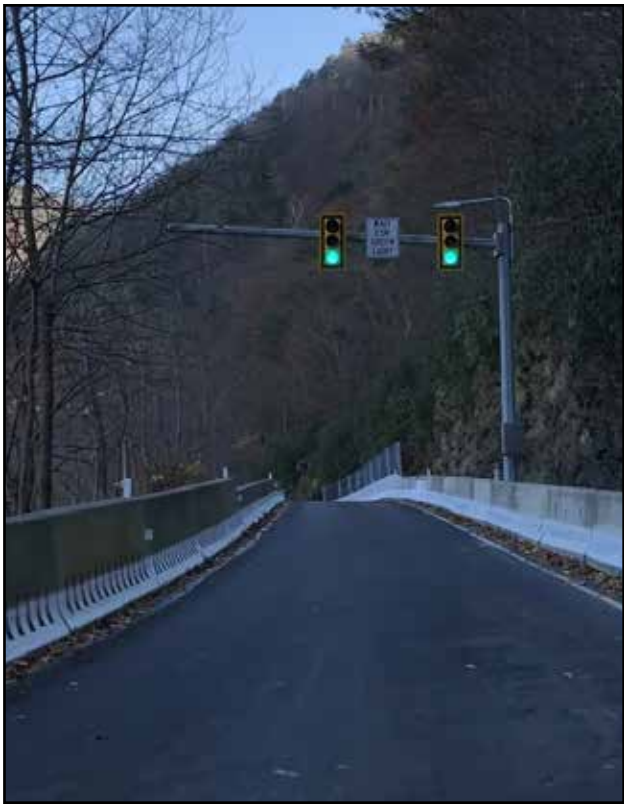
After being closed for almost two years, Route 611 in Delaware Water Gap and Upper Mount Bethel Township reopened on Tuesday, Nov. 5, 2024. Part of the road is one-lane for now. A motorcyclist heading north into the one-lane section waits on the light to change near the Point of the Gap Overlook. Drivers heading north into the one-lane section wait on the light to change near the Point of the Gap Overlook. A driver heading north into the one-lane section waits on the light to change near the Point of the Gap Overlook. Photo by Bob Halberstads/The Free Weekly Press
